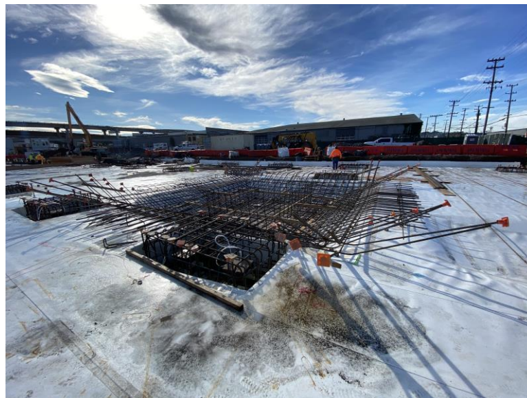
Waterproofing and Rebar at Elevator Pit – December 31, 2019
