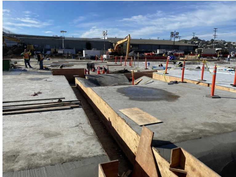
Mud Slab and Underground Utility Trench – December 31, 2019
