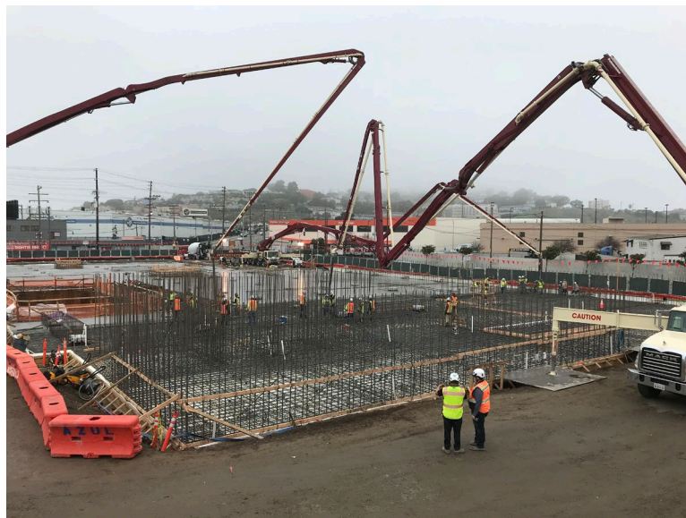
Concrete Pour--Mat Foundation Slab – January 25, 2020
