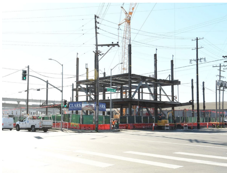
Structural Steel Erection – February 6, 2020
