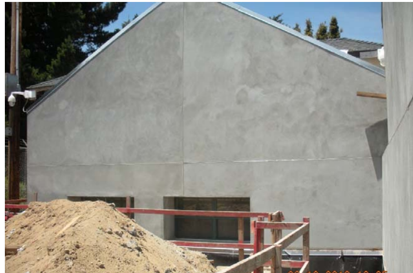
Park Police Station – Shotcrete Shear Wall at South Elevation June 10, 2019
