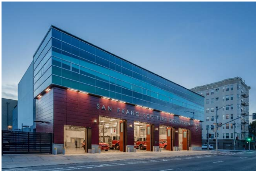
Fire Station No. 5 – Completed April 29, 2019
