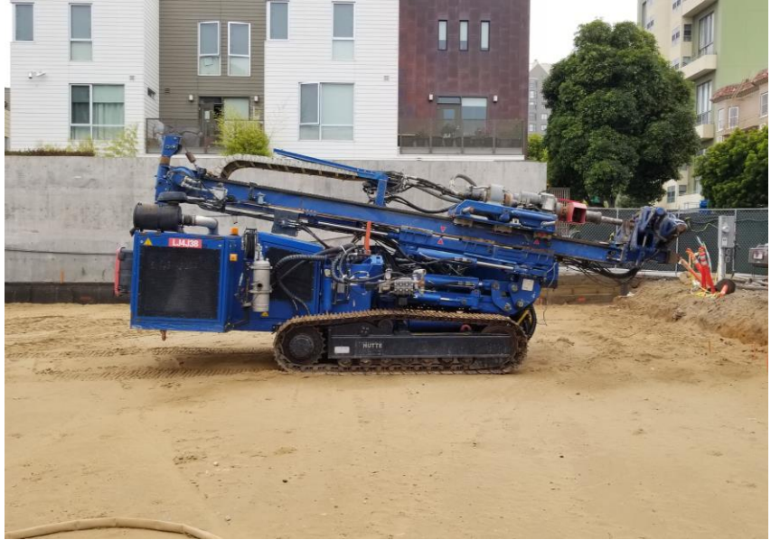
Arrival of the Hydraulic Drill Rig (August 8, 2017)
