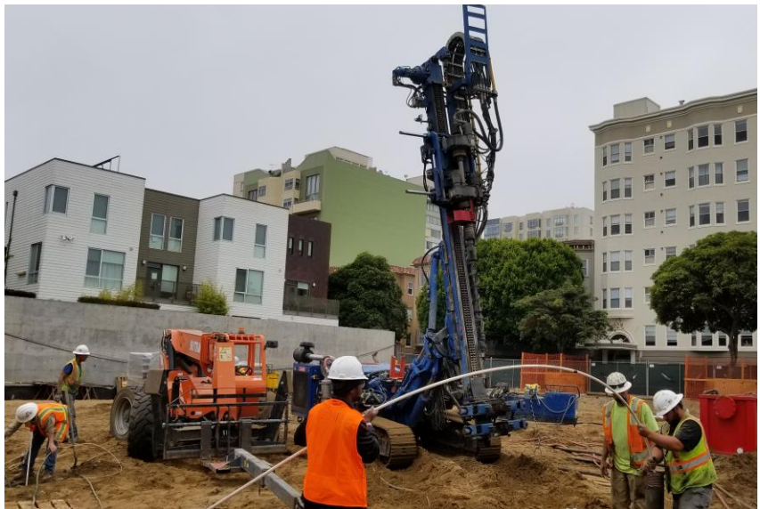
Drilling and Placement of Soil Micropiles (August 15, 2017)
