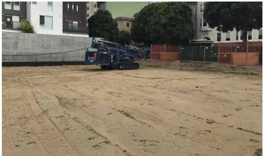
Building Pad is ready to go! (August 4, 2017)
