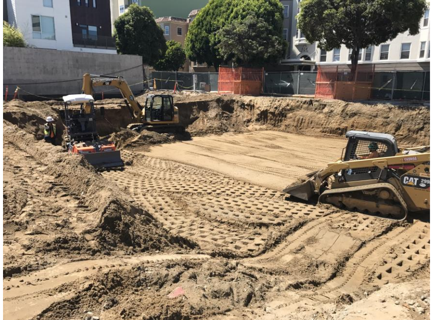
Excavation and Compaction Activities (July 24, 2017)
