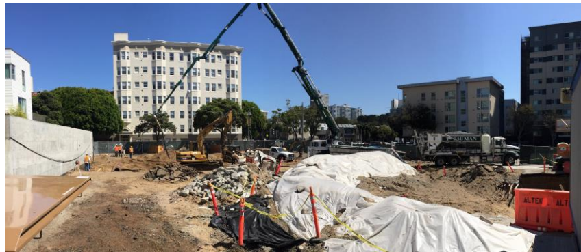
Shoring – Concrete Pour for Soldier Beams (July 19, 2017)
