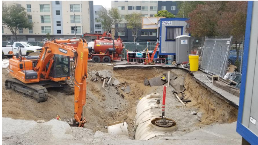
Excavation of final underground fuel storage tank (June 27, 2017)
