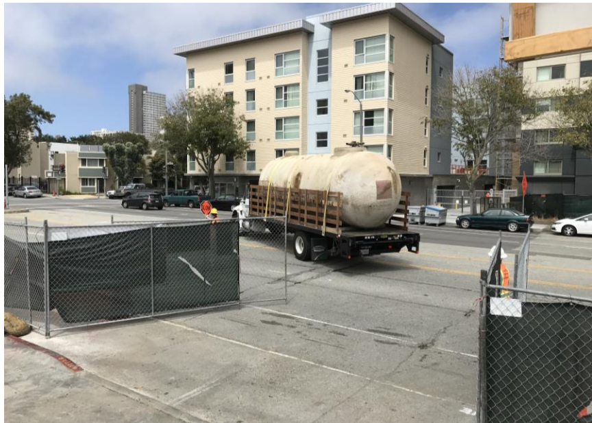
Final underground fuel storage tank being off-hauled (June 29, 2017)
