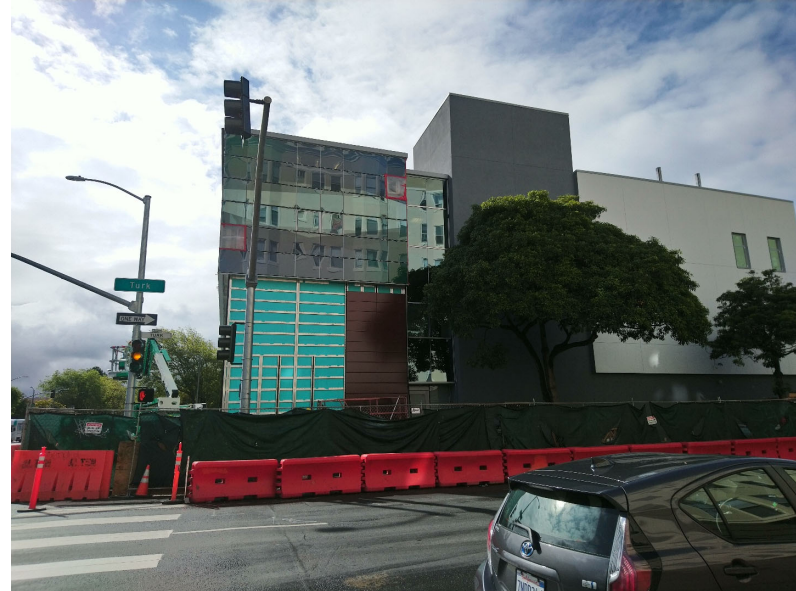
Terracotta Tile Panels at North Elevation (March 1, 2019)
