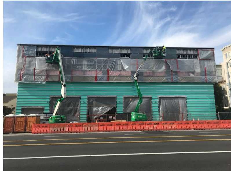
Glass Installation at East Elevation (February 8, 2019)
