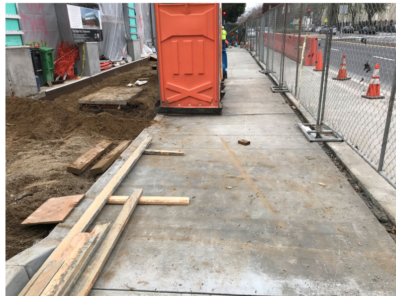
Concrete Curb and Apron at Webster Street (December 20, 2018)
