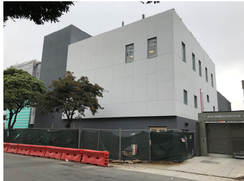
Plaster and Windows at North and West Elevations (December 20, 2018)
