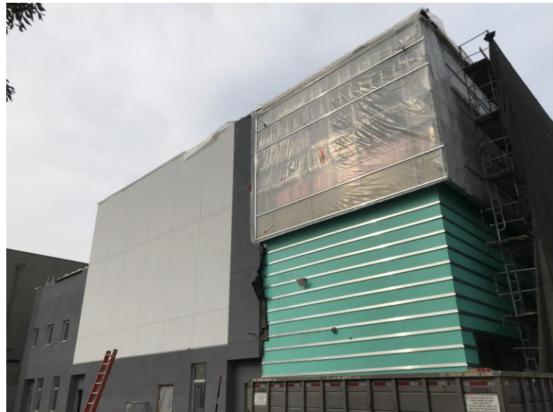
Plaster at South Elevation (November 19, 2018)
