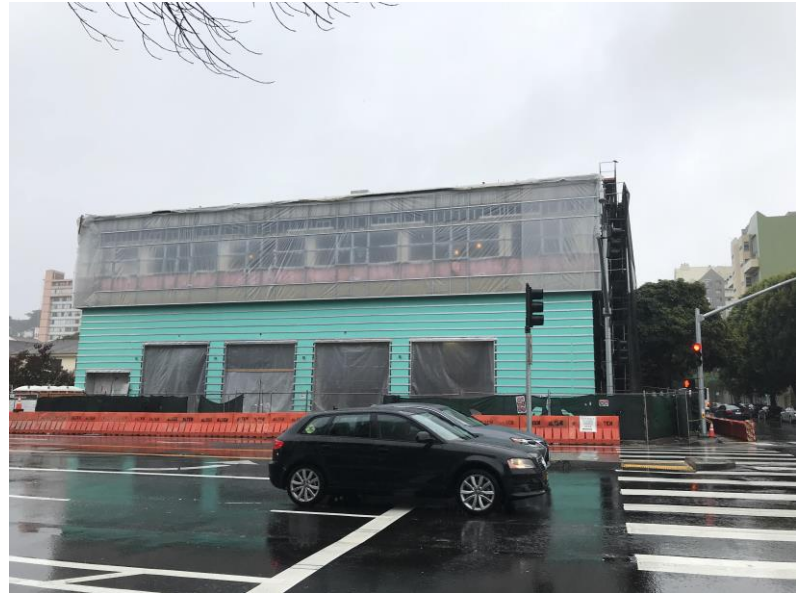
Removed Scaffolding at East Elevation (November 21, 2018)
