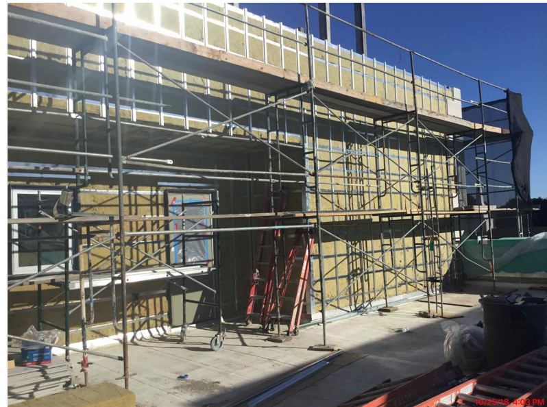
Mineral Wool Insulation at 3rd Floor Terrace (October 25, 2018)
