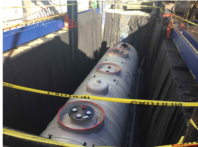
Underground Storage Tank Set at Parking Lot Area (October 25, 2018)
