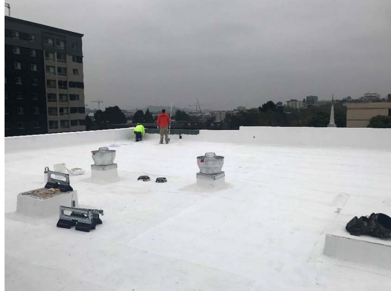
Liquid-Applied 'Cool Roof' (August 23, 2018)
