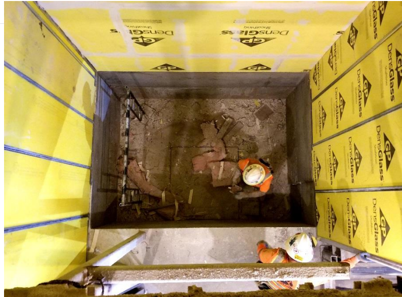
Removing Scaffolding from Elevator Shaft (July 24, 2018)
