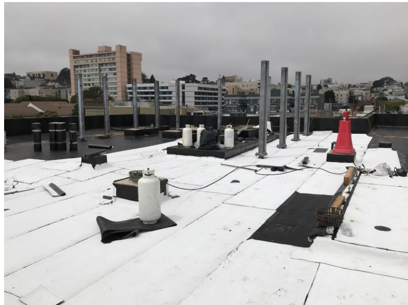
Installation of APP Cap Sheet at Roof (July 24, 2018)
