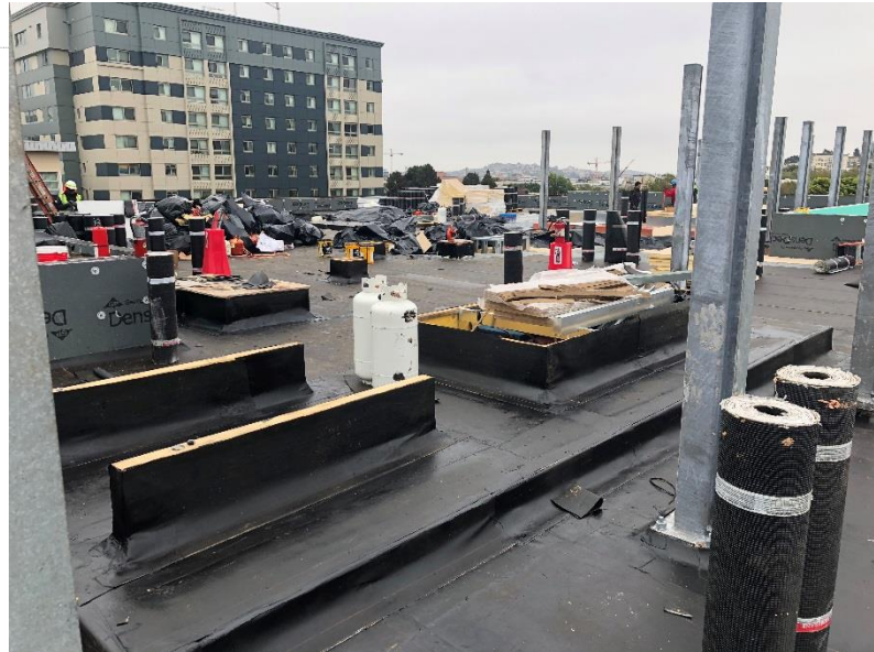
Installation of Fluid-Applied Roofing System (July 12, 2018)
