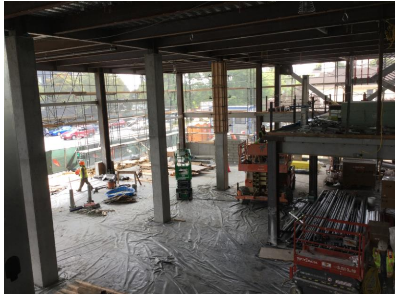
Concrete Encased Steel Columns at Apparatus Bay (April 26, 2018)
