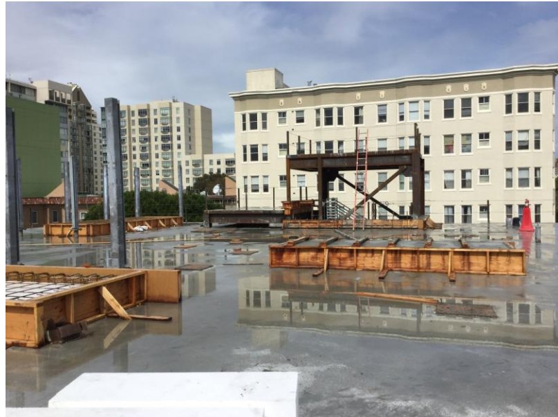
Concrete Roof Deck and Equipment Curbs (March 13, 2018)
