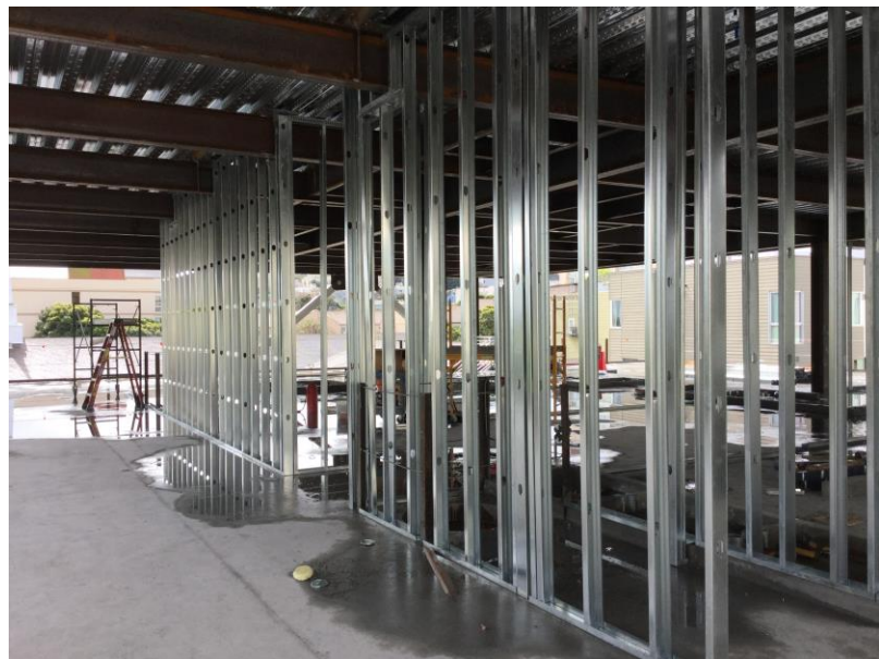
Interior Light Gage Metal Stud Framing at 3rd Floor (March 13, 2018)
