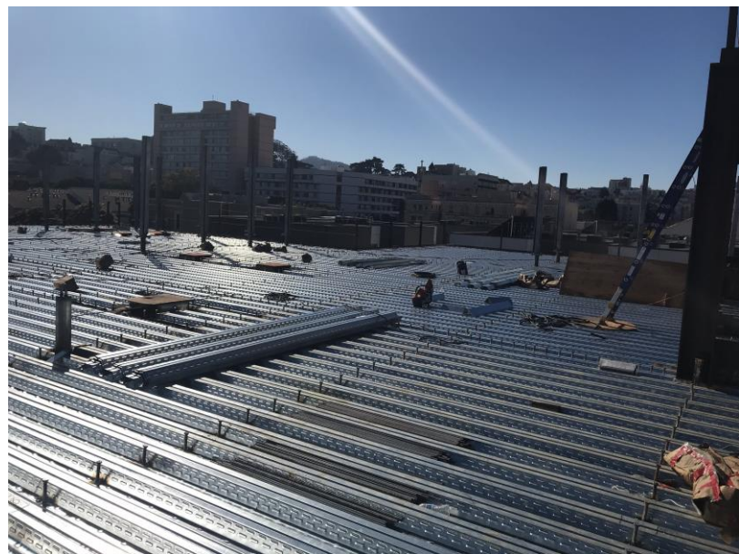
Metal Decking at Roof Level (February 8, 2018)
