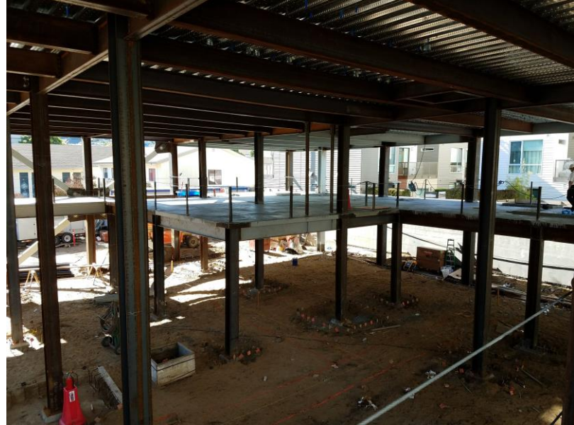
Concrete Slab at 2nd Floor (February 6, 2018)
