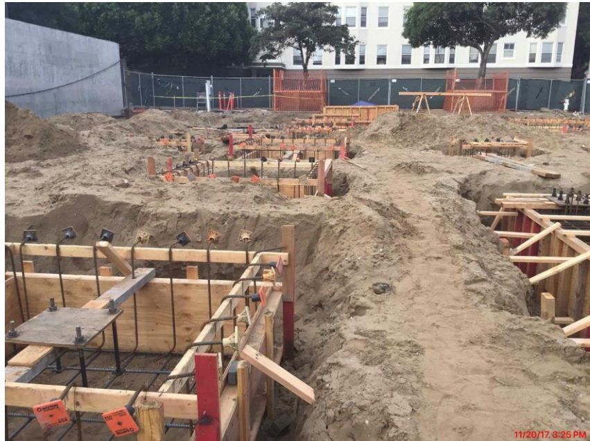
Formwork, Rebar, and Anchor Bolt Placement at Spread Footings (November 20, 2017)
