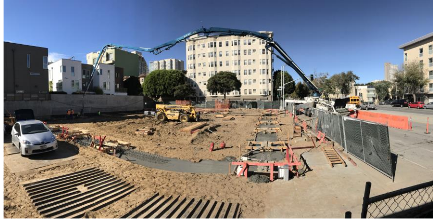
Concrete Pour of Continuous Footings (October 23, 2017)
