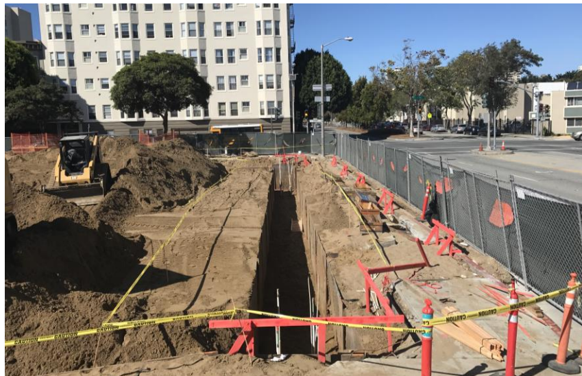
Trenching along Webster Street for concrete footings (September 22, 2017)
