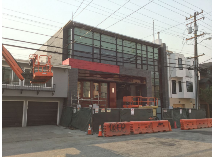
Installation of Stone Veneer Panels at North Elevation (November 9, 2018)
