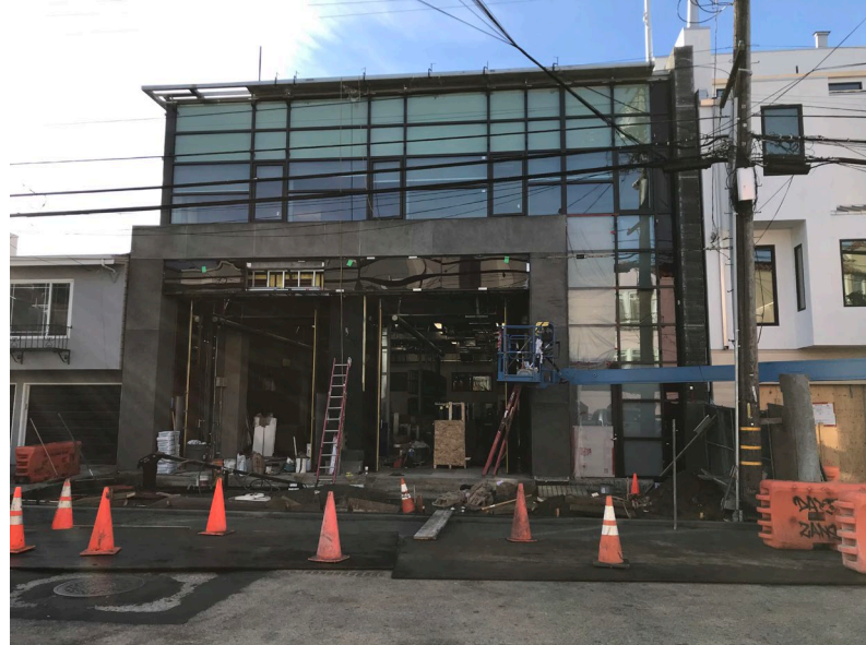
Concrete Apron Placement at Greenwich Street (October 26, 2018)
