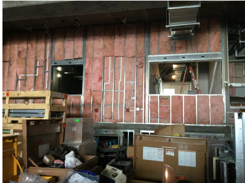
Wall Insulation in the Apparatus Bay (April 13, 2018)
