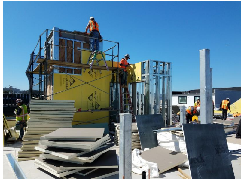
Sheathing Exterior Walls at Stair & Elevator Tower at Roof Level (March 28, 2018)
