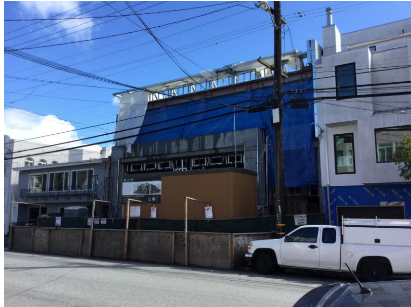
View of North Elevation from Greenwich Street (March 14, 2018)
