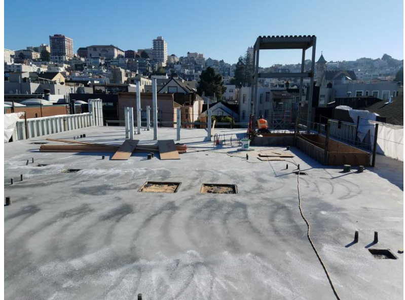
Concrete Deck at Roof Level (February 7, 2018)
