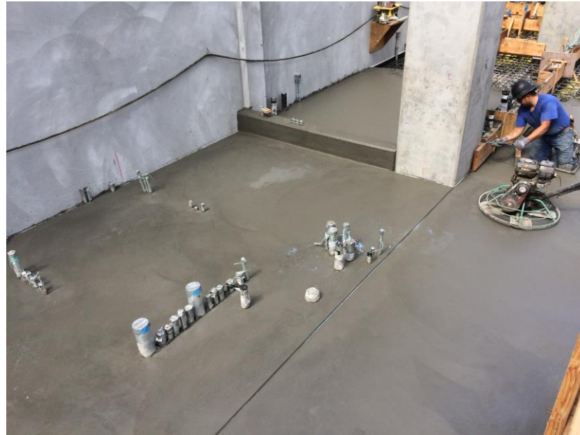
Placement of Concrete Slab at 1st Floor Lower Level (September 20, 2017)
