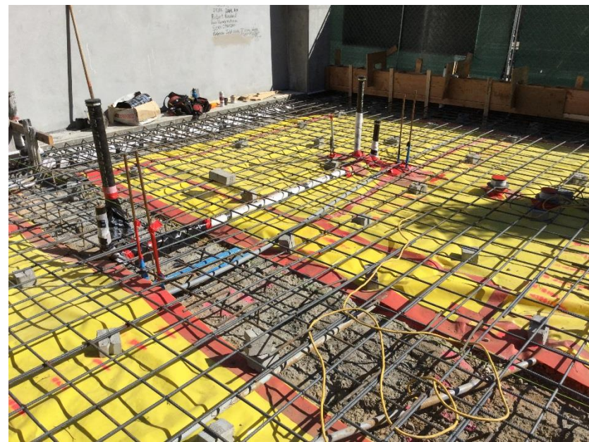
Rebar Installed for Concrete Pour at 1st Floor Upper Level Slab (October 5, 2017)
