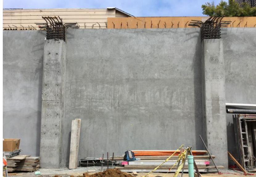
East elevation after 7/31 shotcrete placement (August 10, 2017)
