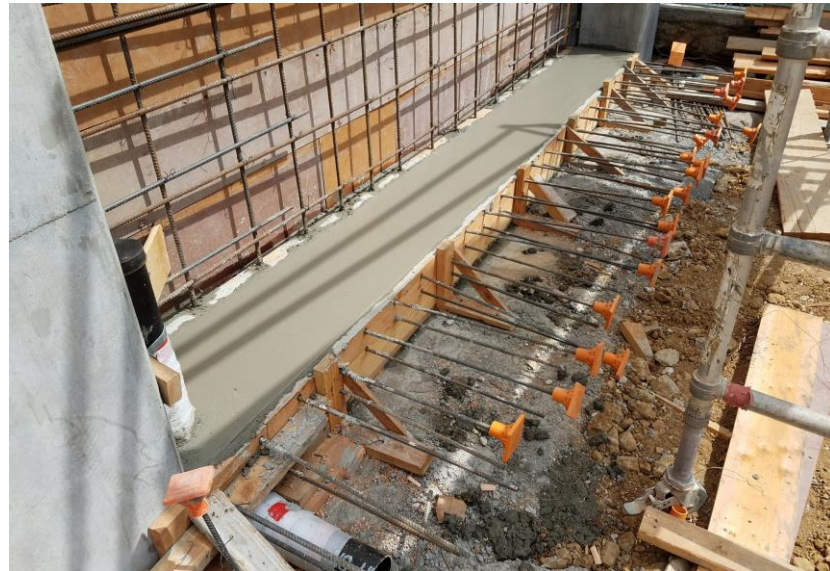
Partial concrete pour at 1st floor upper level slab (August 10, 2017)
