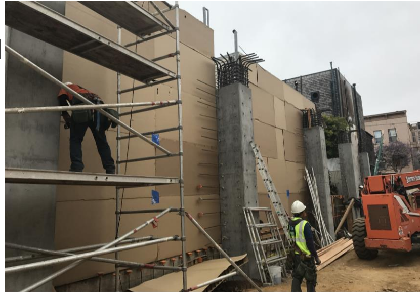
Installation of East wall formwork.
