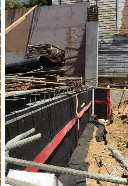
Waterproofing at 1st floor retaining wall.
