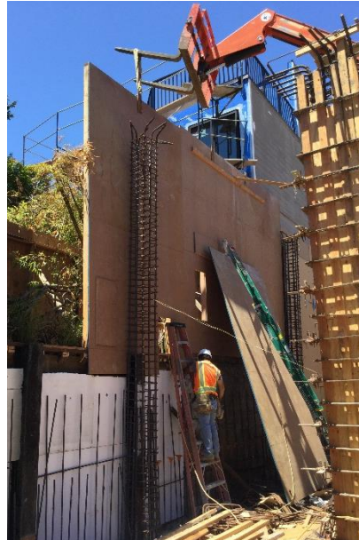
Installation of formwork at West elevation.
