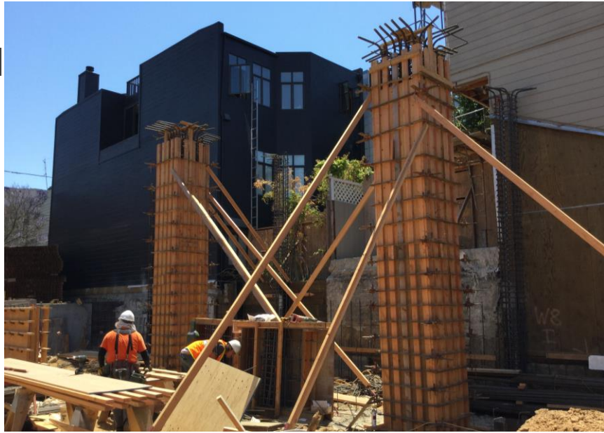
Preparing for pour day scheduled for Thursday, 6/29!
