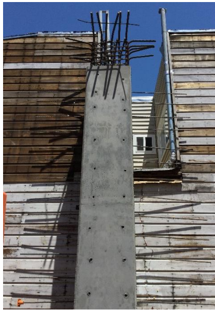
Formwork stripped from placed concrete columns.
