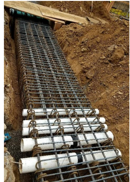
6/8/17: Rebar placement for grade beam at Greenwich Street elevation.
