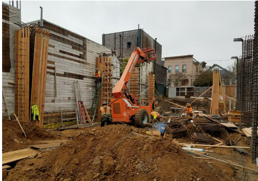
6/8/17: Hard at work preparing for 1st floor columns' concrete pour on 6/14!
