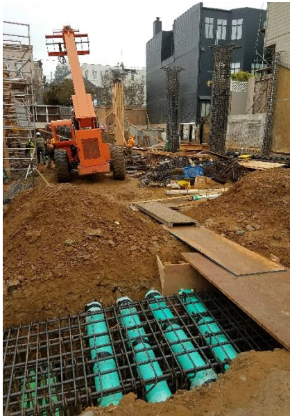
6/8/17: Placement of sleeves for underground utilities.
