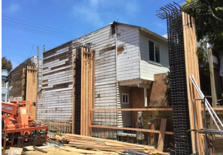
6/1/17: Installation of column formwork in the future Apparatus Bay.
