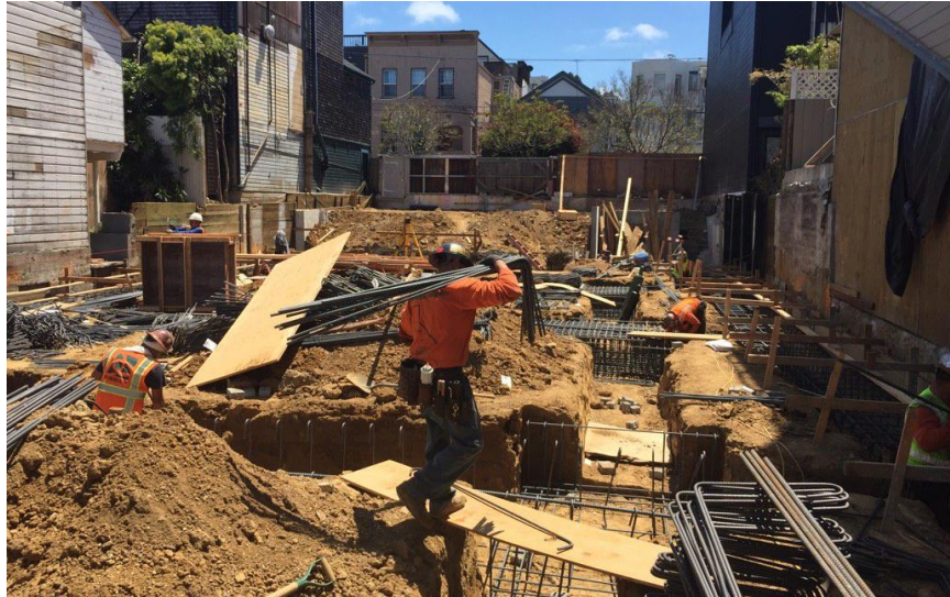
5/11/17: Rebar placement for moment frames and footings.
