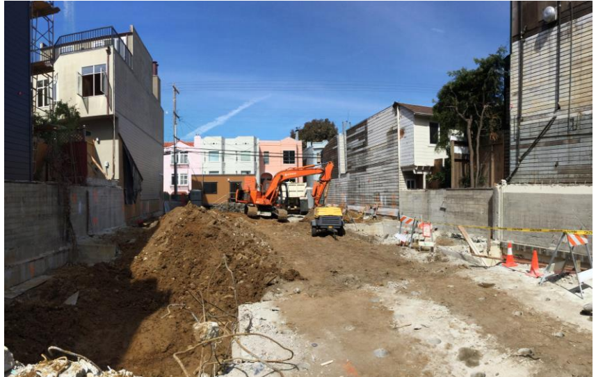
Excavation work and preparation from shoring and underpinning (03.16.2017)
