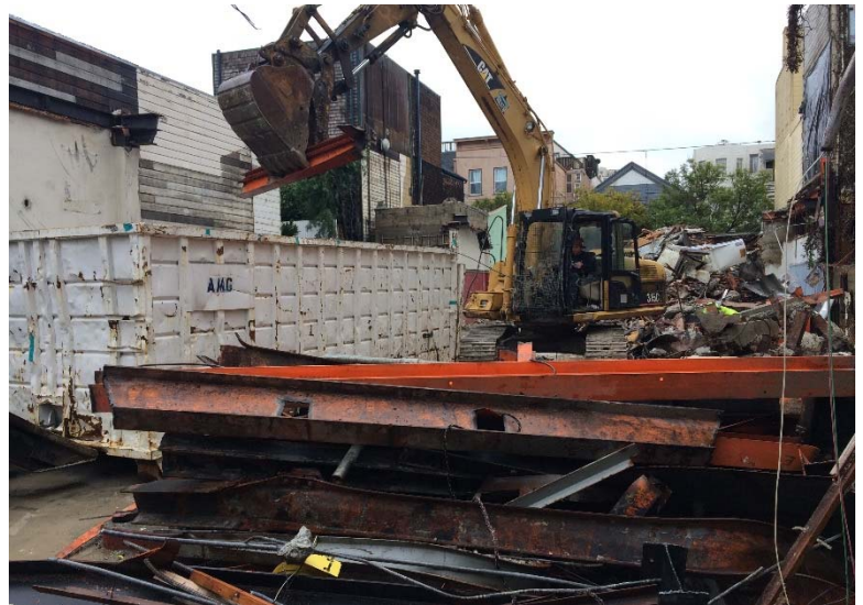
Site separation of demolition debris for recycling.
