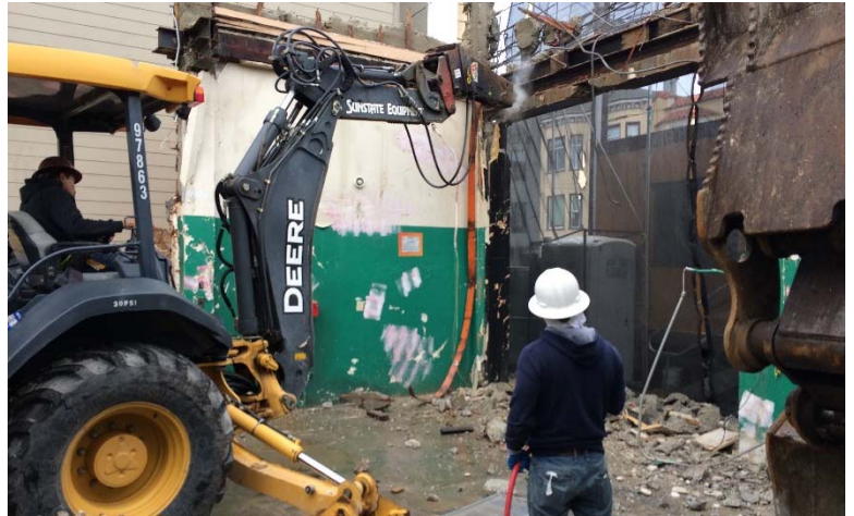
Demolition of the final wall facing Greenwich Street (02.10.2017)
