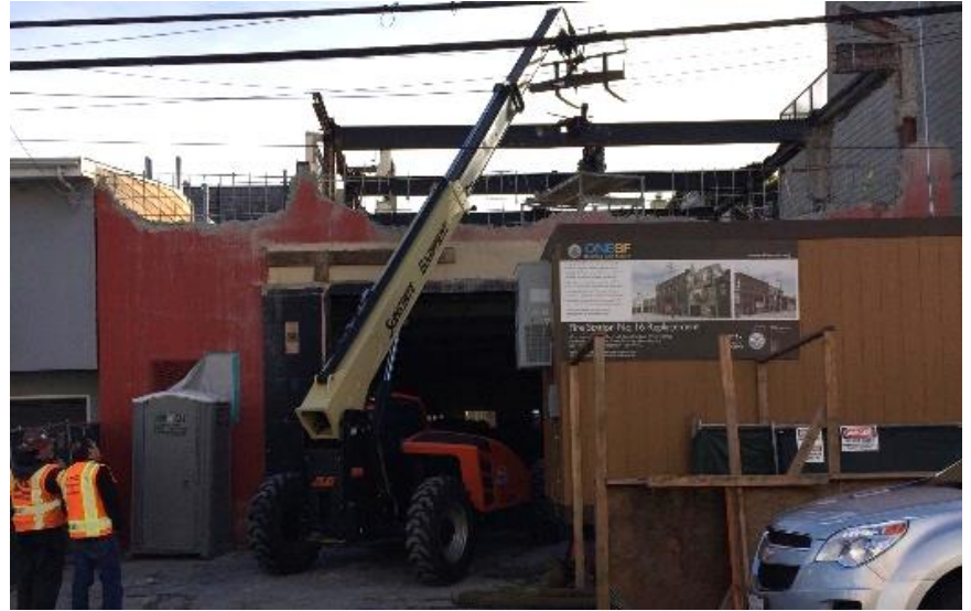
Demolition of structural steel at the roof and 2nd floor using a boom lift (01.06.2017)
