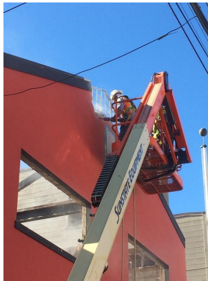
Demolition of front façade facing Greenwich Street (11.17.16)
