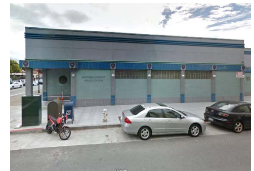
Northern Police Station
