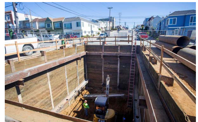
Cistern under construction
