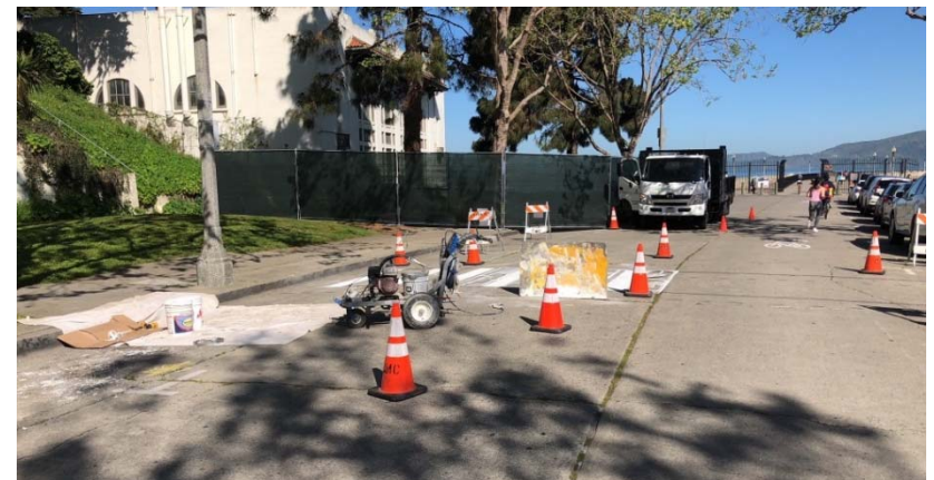
Pump Station 2 Project
