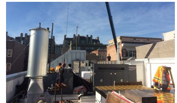
FS 3 Installation of Generator at Roof
