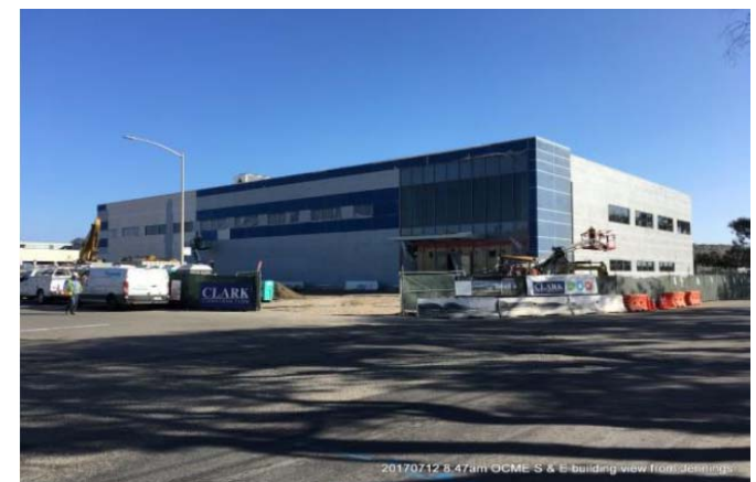
OCME South East Bldg . Entry View
