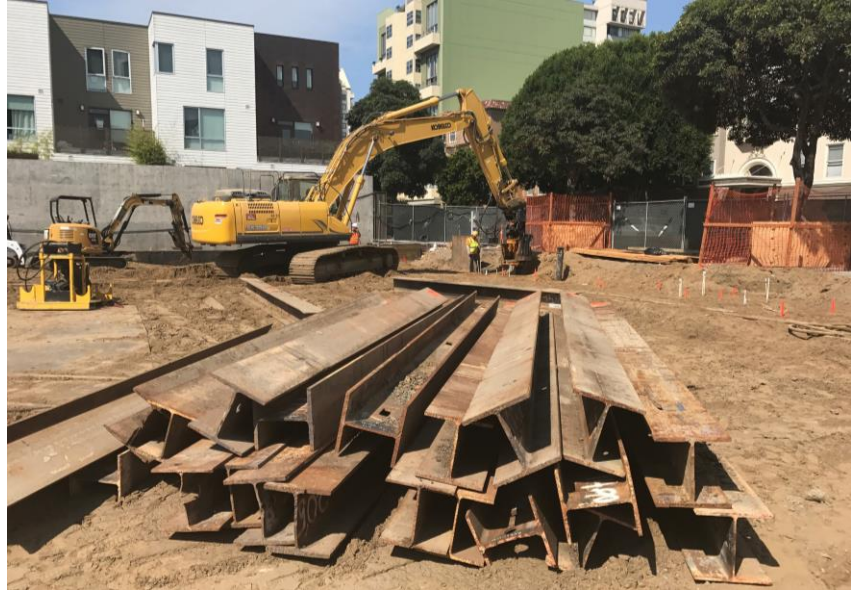
Steel Soilder Beams for Temporary Shoring System (September 11, 2017)
