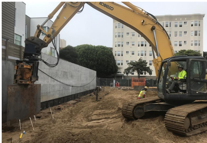
Installation of Steel Sheets for Temporary Shoring System (September 12, 2017)
