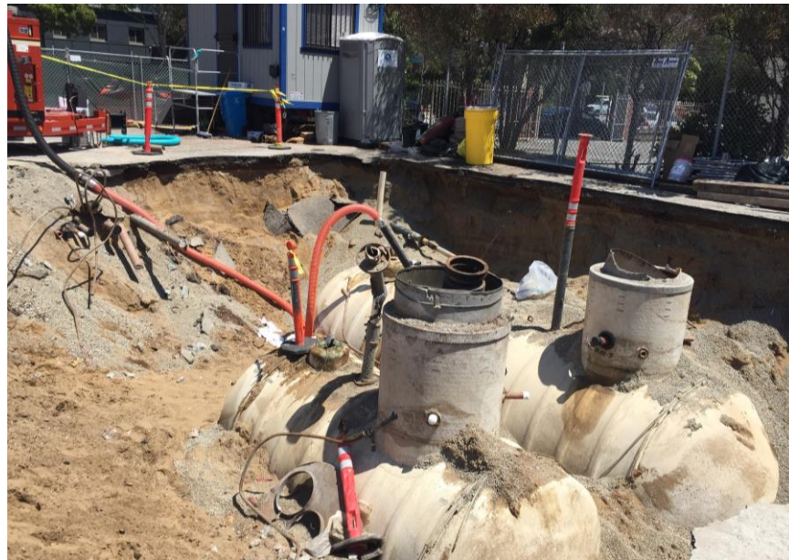
Excavation of underground fuel tanks (June 22, 2017)
