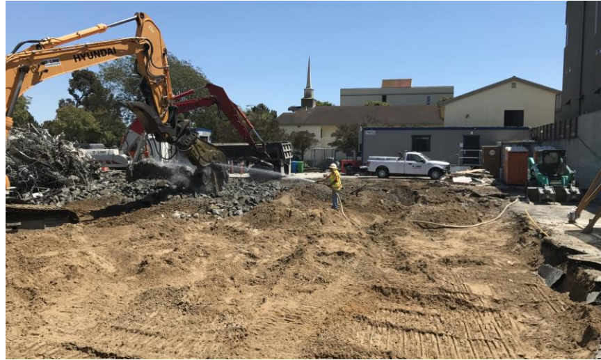
Building demolition complete (June 19, 2017)
