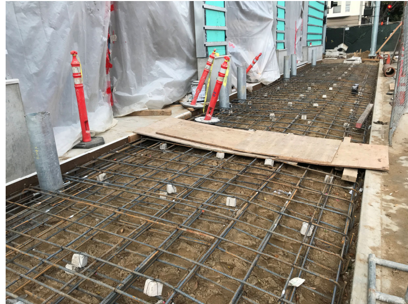
Rebar at Driveway and Sidewalk on Webster Street (January 11, 2019)
