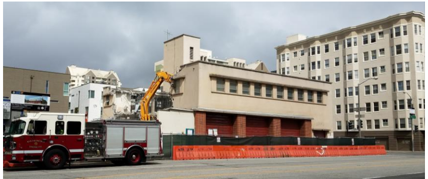
Building Demolition, Day 3 (May 25, 2017)
