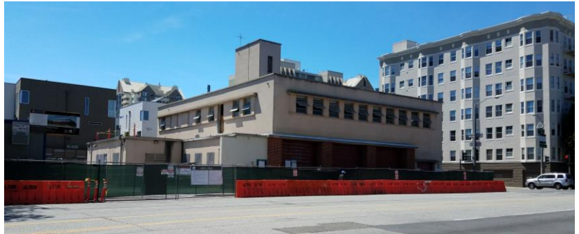
Pre-Building Demolition (May 22, 2017)
