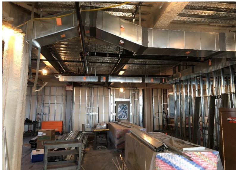
Metal Stud Framing and MEP Rough-In at 1st Floor – Complete (August 6, 2018)
