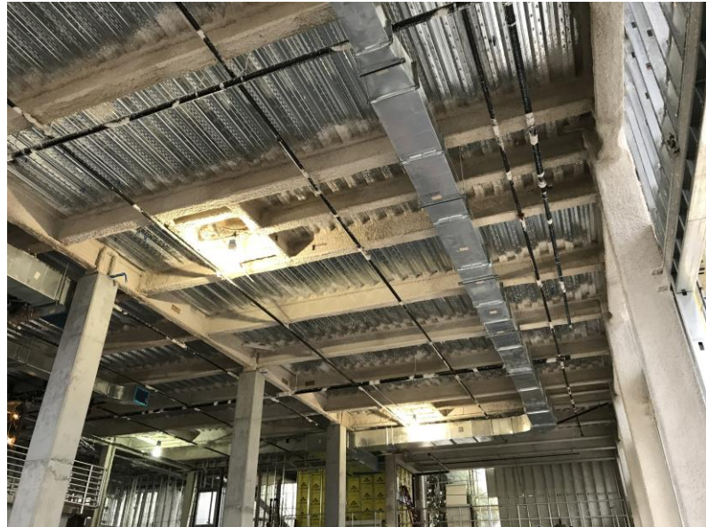
Fireproofing Steel and HVAC Installation in Apparatus Bay (May 22, 2018)
