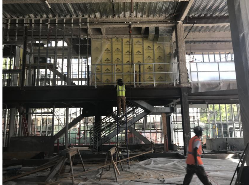
Installing Galvanized Steel Guardrails at 2nd Floor (May 9, 2018)
