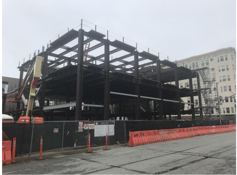
Southeast View from Webster Street (January 11, 2018)
