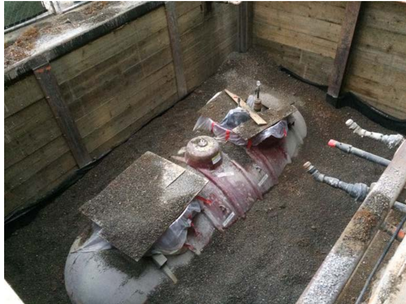
Underground Storage Tank at Greenwich Street (September 18, 2018)
