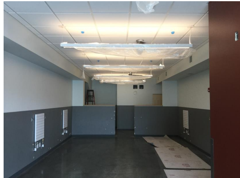
Acoustical Ceiling Tiles at 2nd Floor Dormitory (August 28, 2018)
