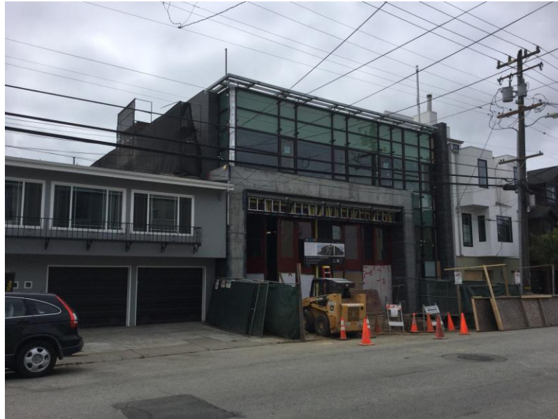
Stone Veneer Tile Panels at East Elevation (August 28, 2018)
